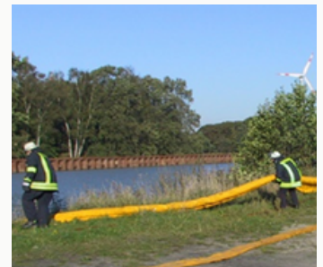
Placing the barrier into the water.
