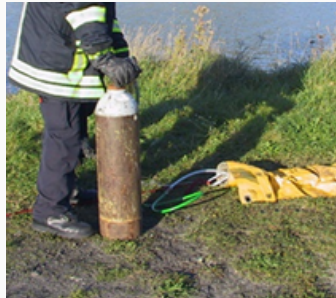
Filling the barrier from a compressed-air cylinder (300 bar).
